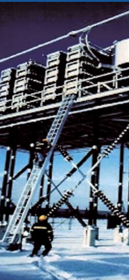
Montagnais 735 kV Series Capacitors bank
