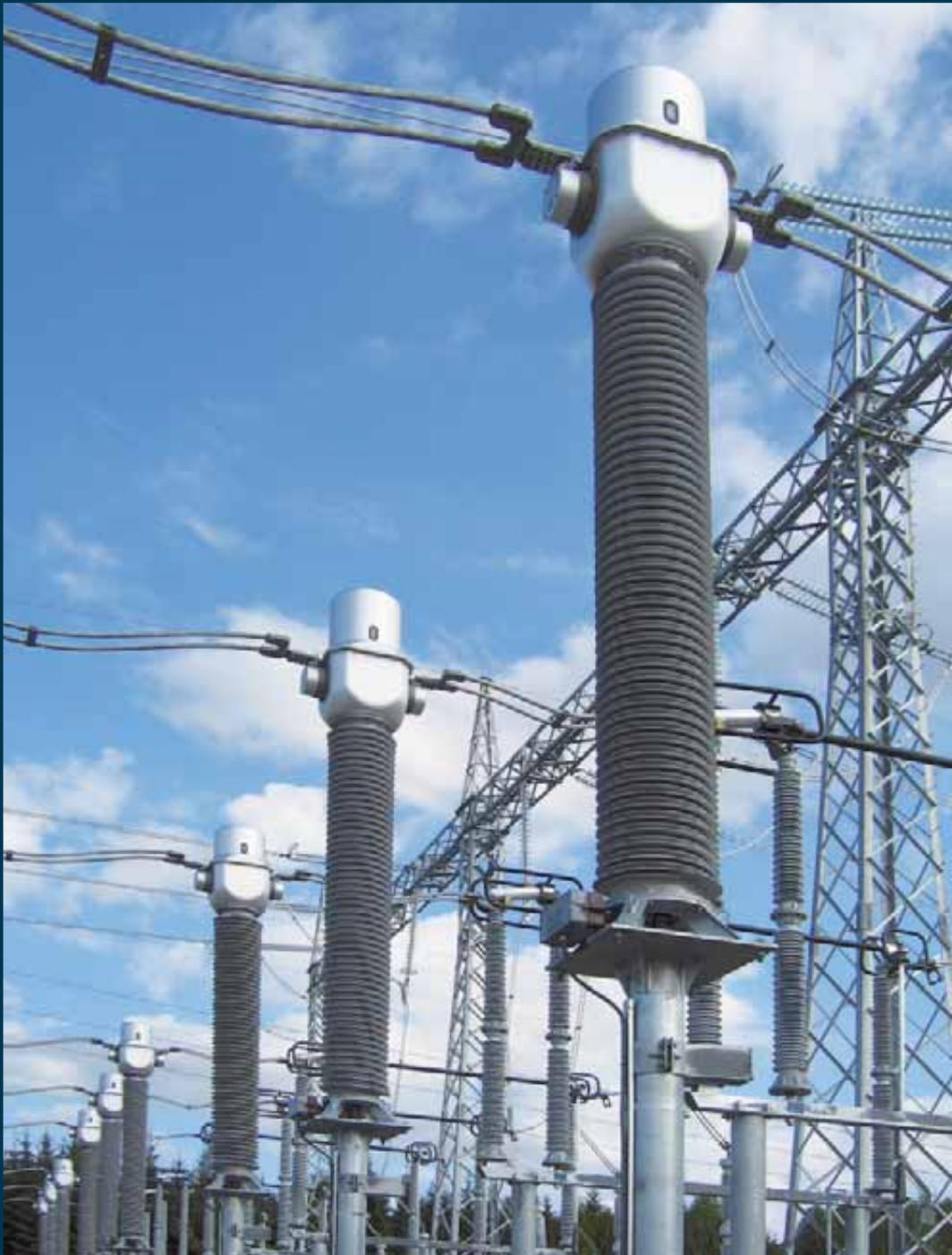
› 420 kV Current transformers with gray silicone rubber insulator. Statnett (Norway).
