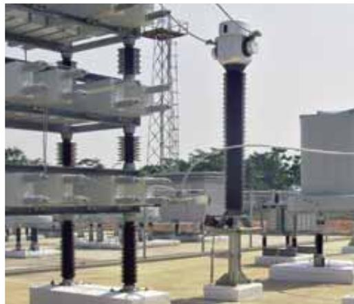
2. 245 kV Current transformer protecting capacitor bank (India).
